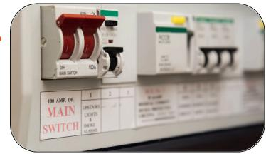
MCBs (Miniature Circuit Breakers) are typically a series of smaller switches marked "lights, sockets, cooker" etc. Simply flip this back to "on" and you should have power.
